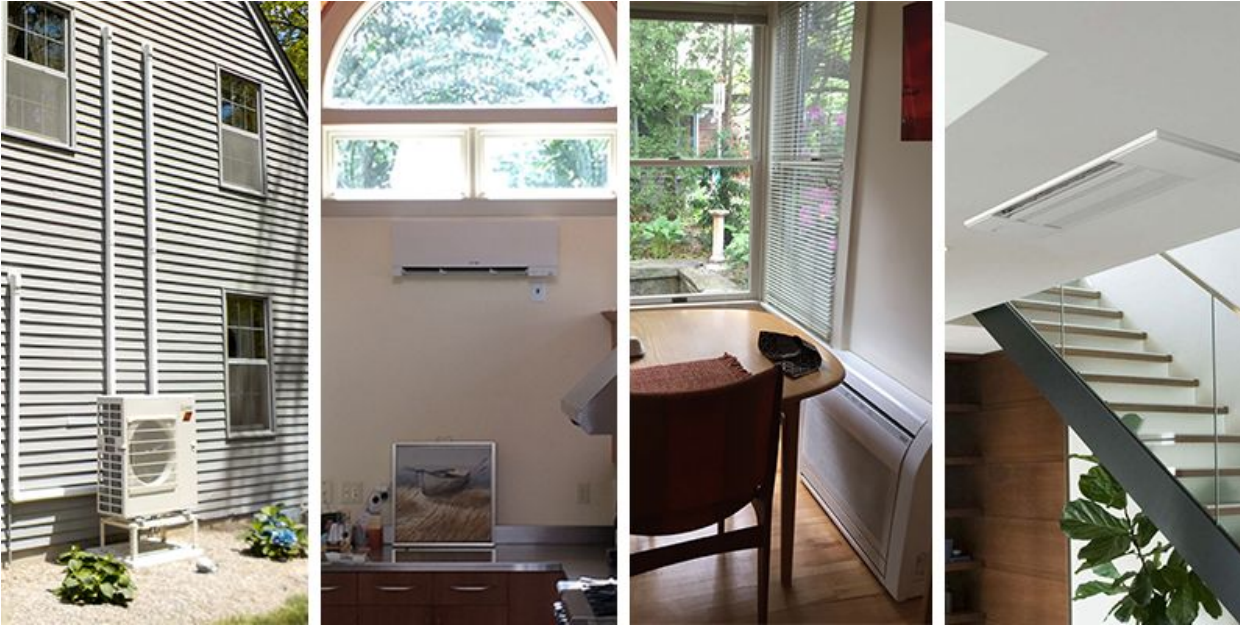
From left to right: (1) a ductless outdoor unit, (2) a standard wall-mounted indoor unit, (3) a floor-mounted indoor unit, and (4) a ceiling cassette indoor unit.
