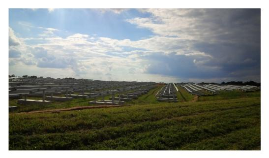
Photo 14: Racking System installation, Parklands Landfill, NJ. Note concrete ballast (Photo courtesy of Waste Management)
